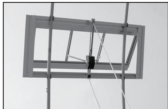
VIEW OF VENT OPEN FROM INSIDE OF GREENHOUSE
